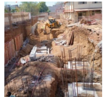
Building under construction
